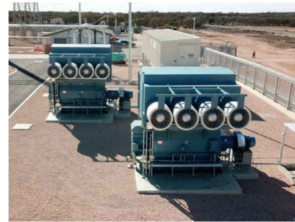
Above: Figures 2a and 2b. Synchronous condensers (left) installed at the Darlington Point solar farm (right) in New South Wales, the largest solar farm connected to Australia's grid
