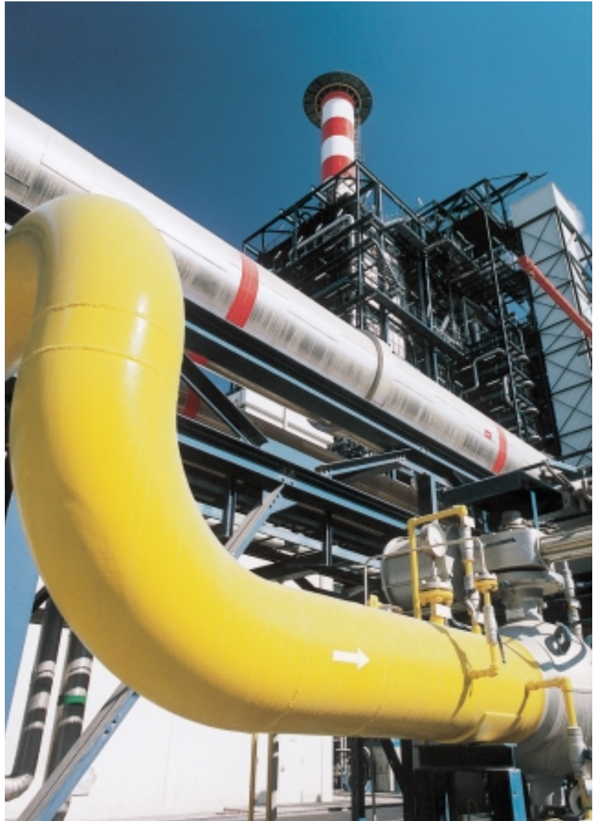
Gas supply line to one of the six steam generators at the Al Taweelah B power plant
