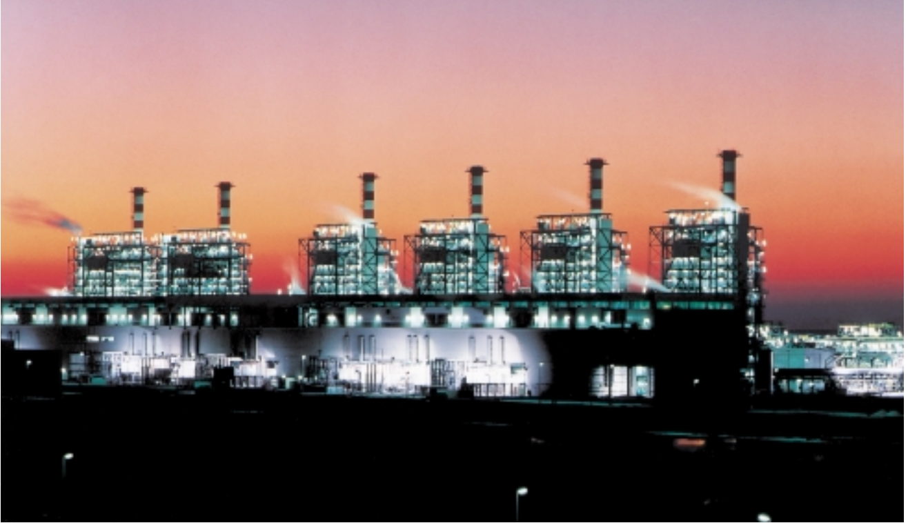
Al Taweelah B steam power station in full commercial operation
