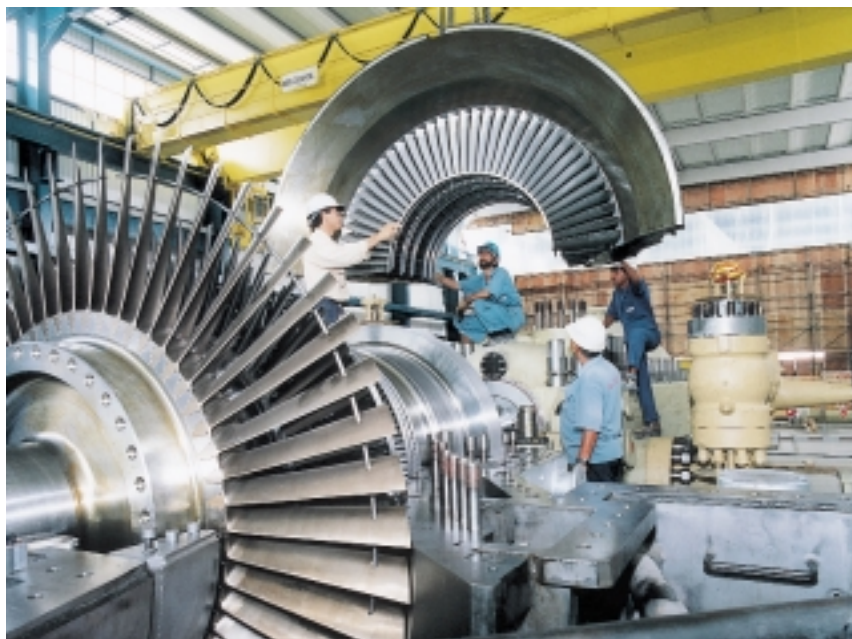
Assembly work being carried out on one of the six steam turbines. Hanging from the crane is the top outer casing of the low-pressure turbine, the last blade row of which can be seen in the foreground.
