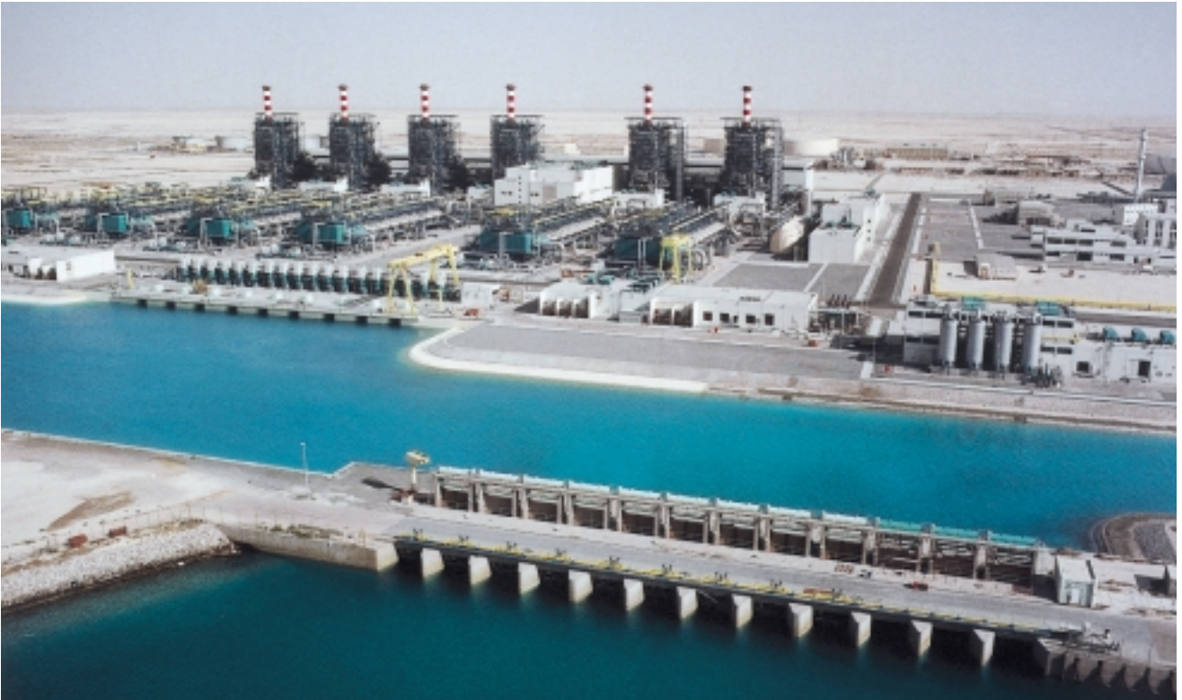
Al Taweelah B steam power plant in Abu Dhabi. Behind the row of pumps in the water inlet pool are the six seawater desalination lines with the interposing control room buildings. The mosque can be seen on the far right, at the height of the six steam generators. 1
