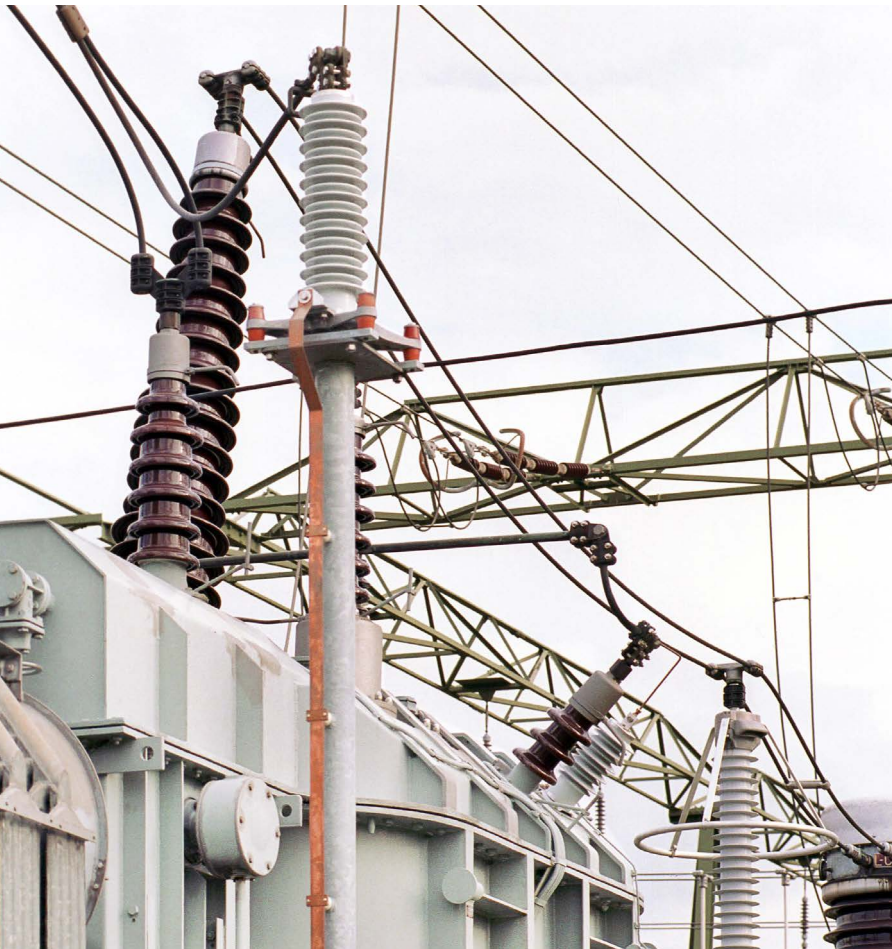
— Overvoltage protection of transformers
