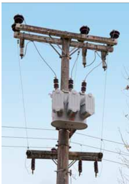
10 An ABB distribution transformer in Brazil
