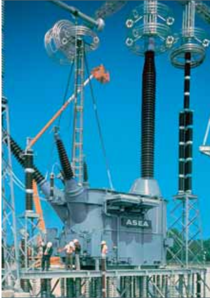
3 The 1785 kV UHV transformer installed at the AEP-ASEA test station outside South Bend, USA. The transformer is installed on an insulated platform to study the effect of line voltages up to 2200 kV phase-to-phase
