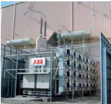
5 One of six converter transformers installed at the receiving end of the Pacific intertie transmission serving the Los Angeles area
