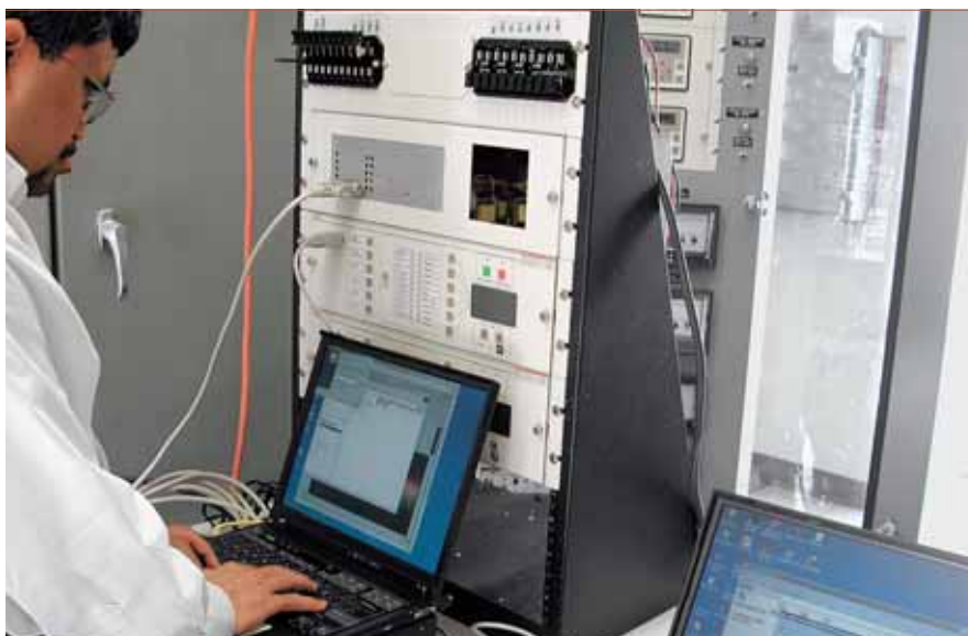
5 IEDs equipped with HIF Detect™ and data collection system
