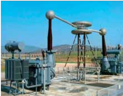
4 1000kV test setup with transformer and shunt reactor at ENEL research station in Italy
