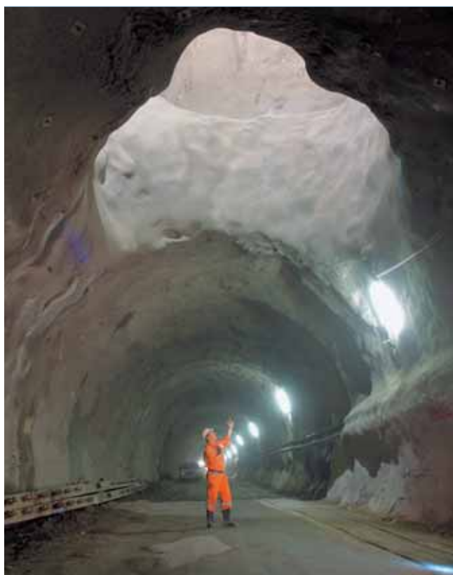
Ventilation tunnel at Sedrun. © AlpTransit Gotthard Ltd
