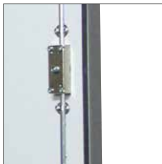
2-point locking using rod lock
