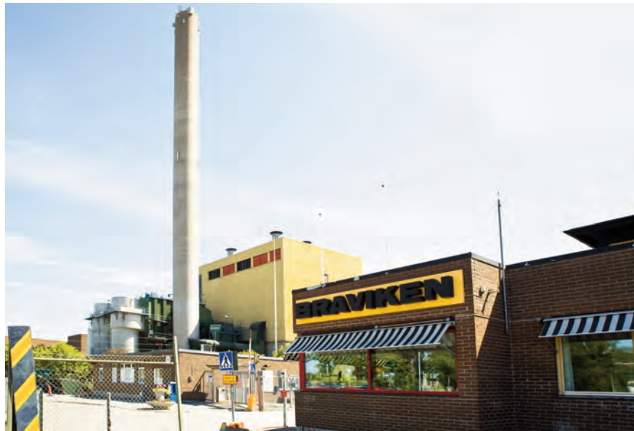
ABB Force Measurement has supplied Holmen Paper AB Braviken, Norrköping, Sweden with, in total, 40 Pressductor PillowBlock Load Cells
