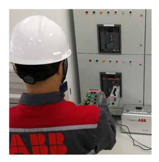
ABB SACE offers a dedicated device to remotely perform circuit breaker rack-in/rack-out operations for SACE Emax 2, increasing the safety for personnel. ABB is constantly committed to the safety of the personnel during every phase of use of its products, including installation and maintenance. During the rack-in operations of the circuit-breaker, the RRD prevents risk of injuries due to possible electric arc.
