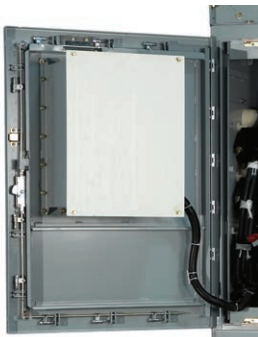
Rear of low voltage box with medium voltage door open
