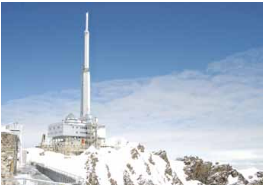
Lightning Protection Group at the Pic du Midi, close to Bagnères de Bigorre in the south west of France
