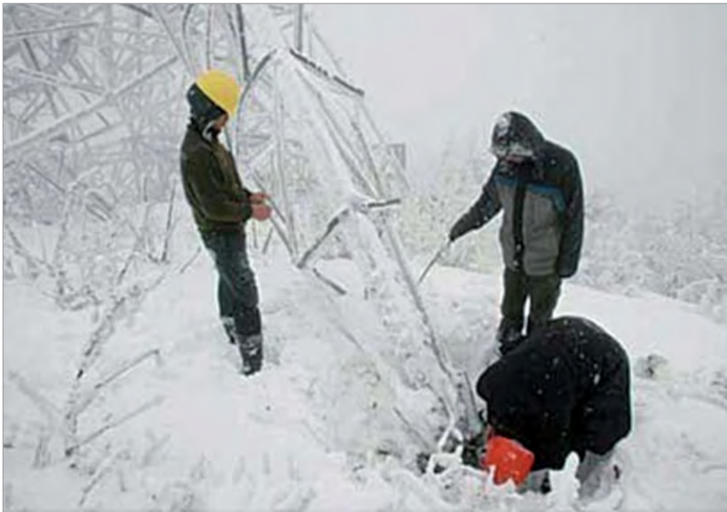
Figure A3 – Ice-damaged transmission tower, China [1]
