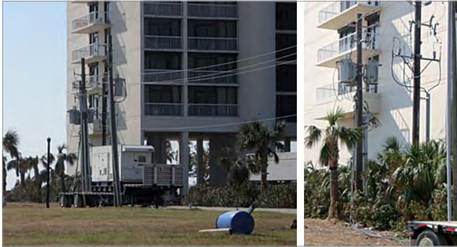
Figure A4-3 – Apartment complex in Galveston Island, Texas, powered by a portable generator connected to the distribution portion of the grid [24]
