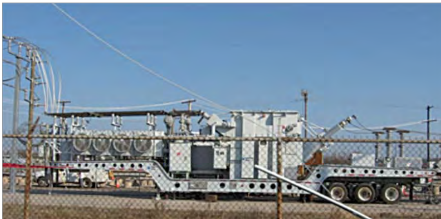
Figure A4-4 – Portable transformer used to restore service in a damaged substation [24]
