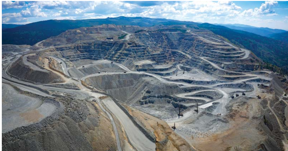
Panoramic view of the Copper Mountain site in British Columbia, Canada. ABB’s Ability eMine trolley system reduced CO 2 emissions on part of the haul route by 90%. (Photo: ABB)
