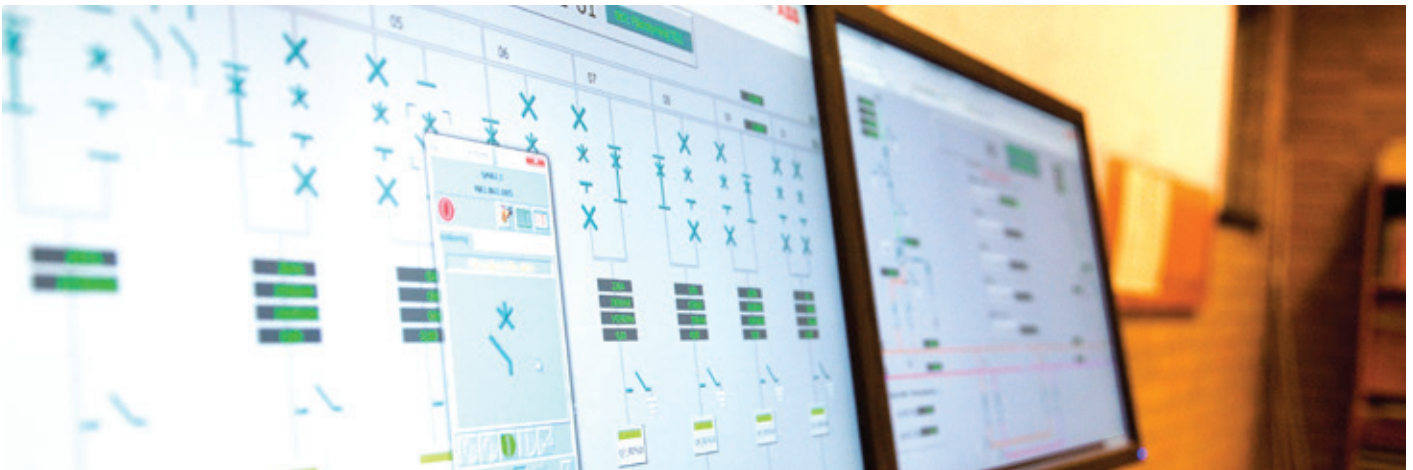
System 800xA provides monitoring and control of electrical equipment in operator control rooms and office environment.
