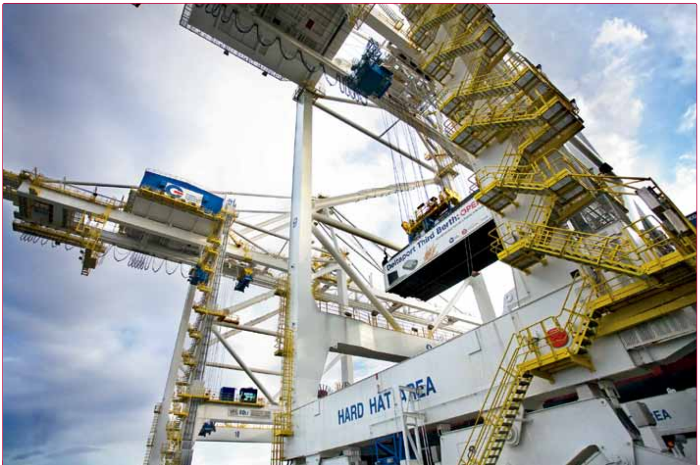
Ship-to-Shore crane with dual hoist
