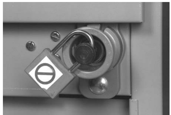
Figure 4.12 Locking the switch disconnecter / earthing switch drive mechanism
