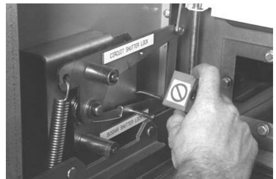
Busbar shutter safety Lock
