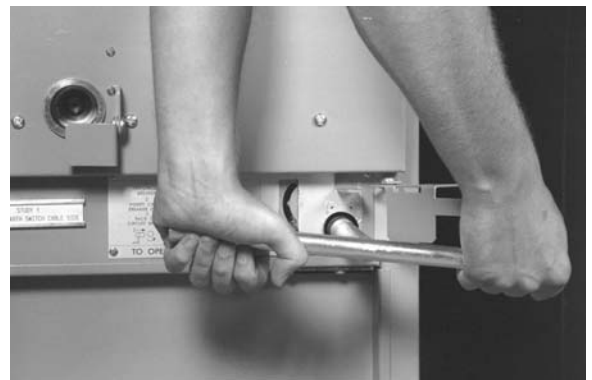
Figure 4.9 Operating the earthing switch
