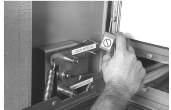
Circuit/cable shutter safety Lock
