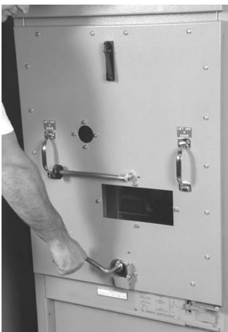
Figure 4.5 Switching device racking
