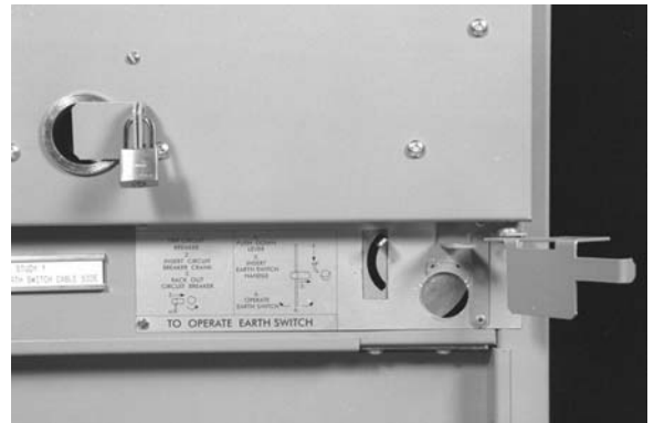
Interlock lever up earth switch drive mechanism not accessible
