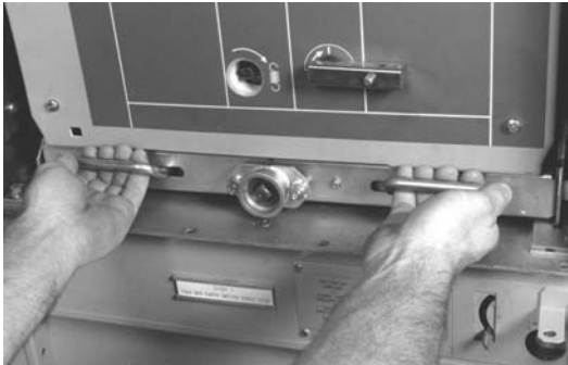
Figure 4.3 Securing/removing the switching device
