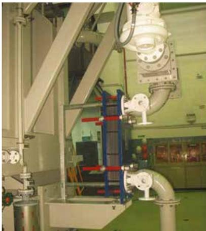
Figure 10. Typical compact ester/water heat exchanger in the underground room
