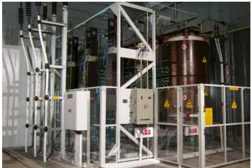
Figure 13. 72 kV dry-type transformer inside of a building (urban substation)
