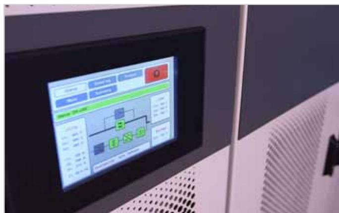
600 kVA PCS100 UPS-I bridges the time between the utility failing and the generator starting
