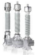
5 Instrument transformers, disconnectors
