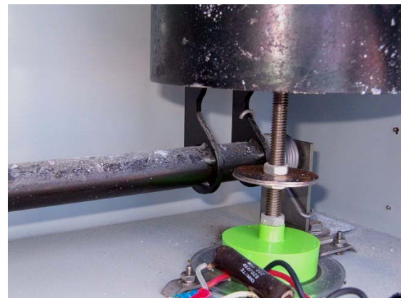
No damage to magnetic actuator assembly
