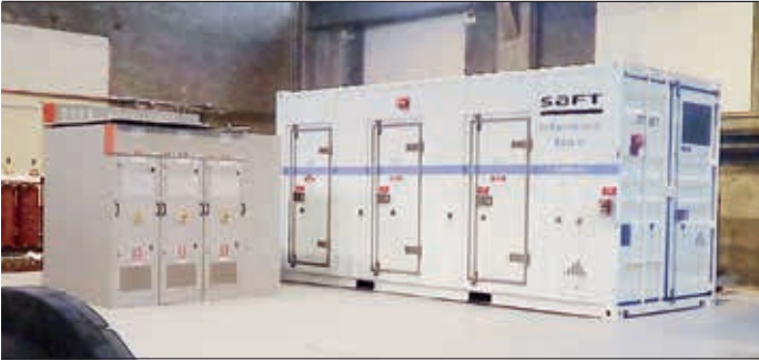
6 ESS batteries and converter cabinets in an installation in Philadelphia, PA, United States
