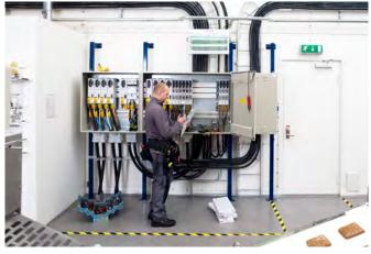
Distribution board in powder coated enclosure mounted on the wall in a switchgear room at a bakery, in Gothenburg, Sweden.
