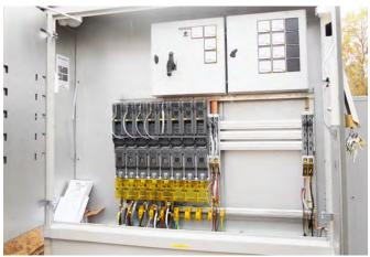
Kabeldon switching devices SLDL, Sweden, especially designed for CSS.
