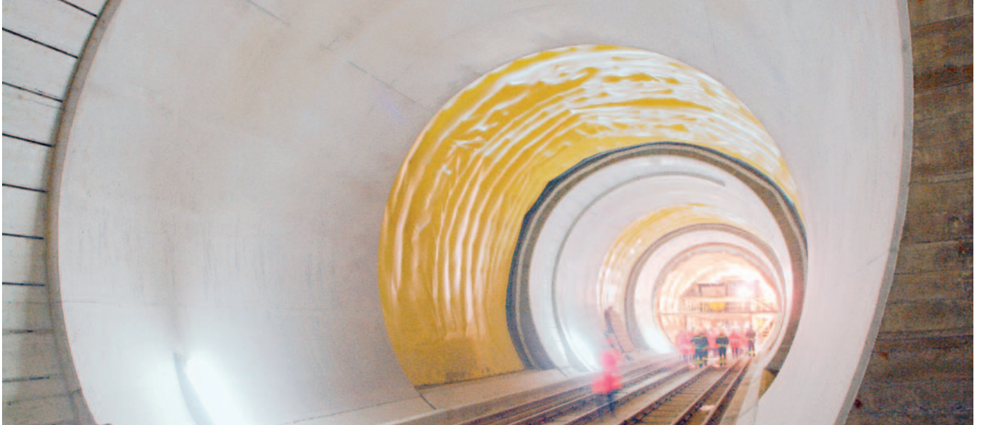
Picture courtesy from AlpTransit Gotthard AG
