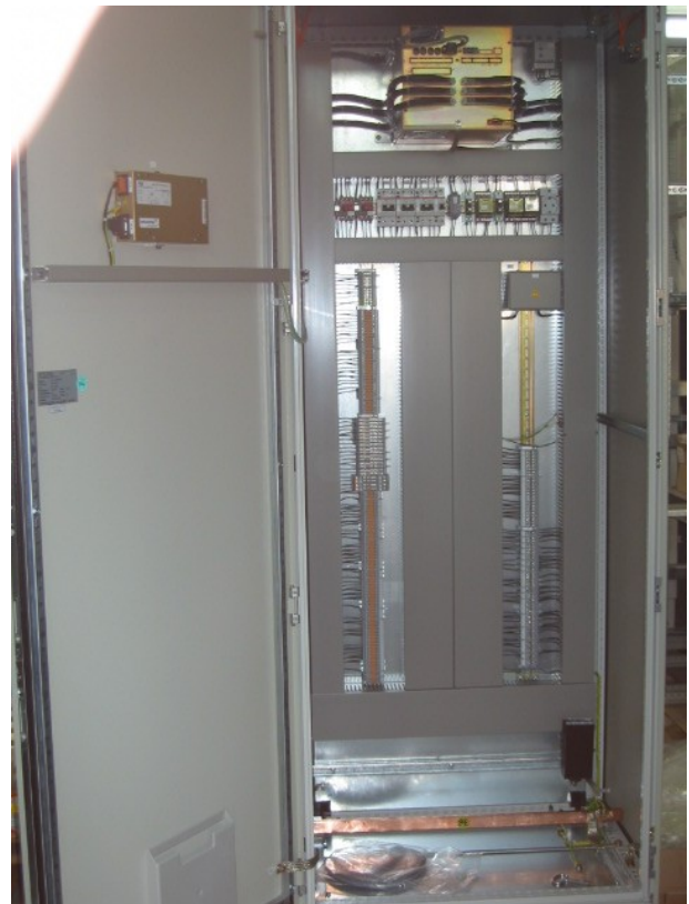
Figure 3-3 High Speed Transfer Device SUE 3000, mounted in a steel sheet cubicle
