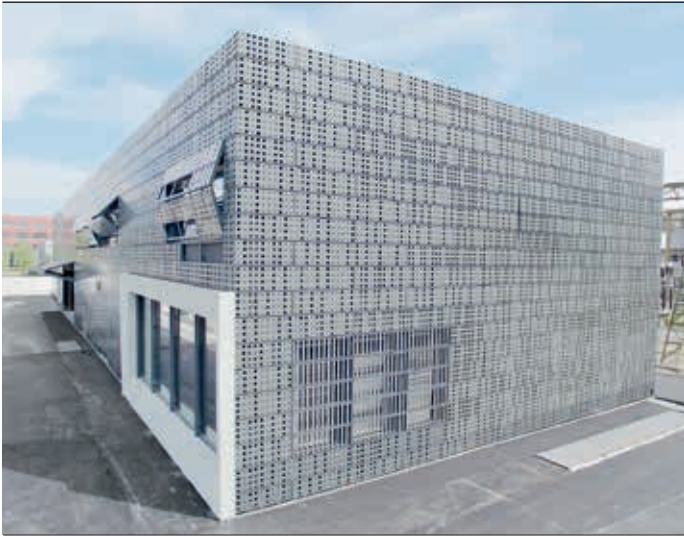
5a The Oerlikon substation building
