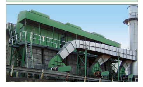
gy audit on filtration plants belonging to Boliden MKM (a leading manufacturer of brass and copper products) by measuring the energy use during a typical production week. The audit mainly covered the fume extraction filter plant for the brass casting process, which consists of two Luhrfilter filtration plants, one with a 250 kW fan and the other with three 132 kW fans **I**. The airflow from the fans was controlled using dampers as restrictors.
