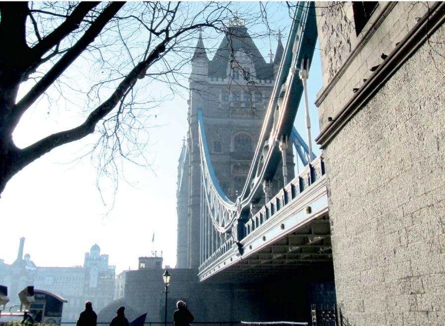
Digital upgrade of ABB load monitoring system helps extend life of London's landmark Tower Bridge. When it was first constructed, Tower Bridge was the largest and most sophisticated bascule bridge ever to be built. The bascules were operated by hydraulics, using steam and giant pumping engines and, despite the complicated procedure, the bascules only took a minute to raise to their maximum angle of 86 degrees.
