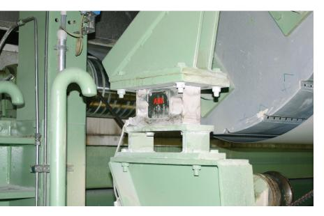
The paper machines and the three coating machines are running with PillowBlock load cells providing an accurate web tension measurement.
