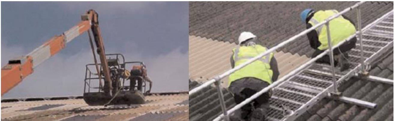
Figs 3 & 4 Examples of safe means of access
