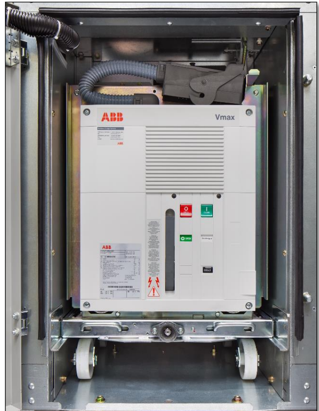
Figure 5: Circuit Breaker in Disconnect Position
