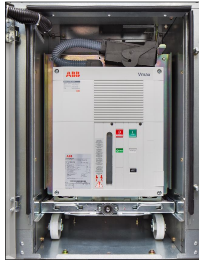
Figure 6: Circuit Breaker in Disconnect Position
