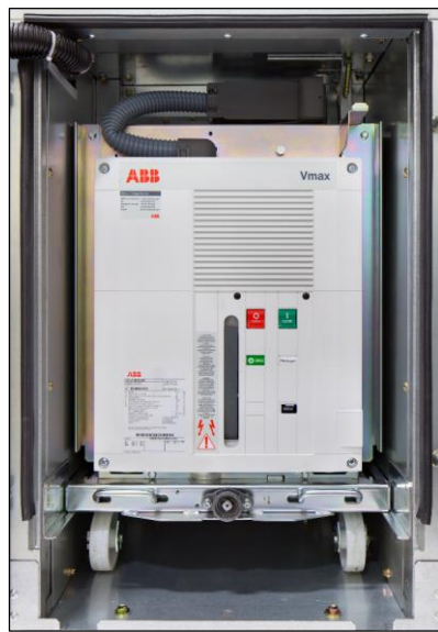
Figure 7: Circuit Breaker in Test Position
