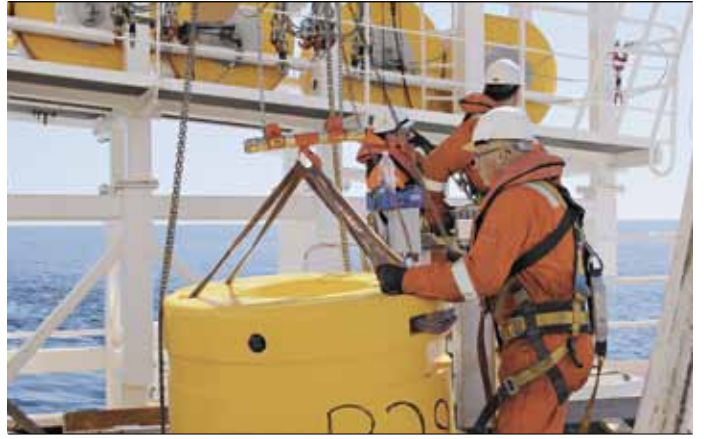
7 One of the buoyancy units used in the lazy wave configuration → 2
