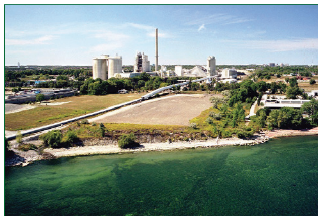
The Mississauga plant.
