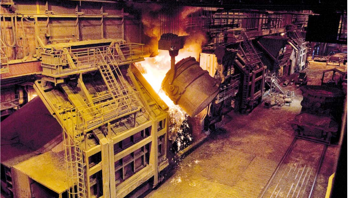
ABB industrial drives with crane control program provide precise control of the 200 tonne charging crane.
