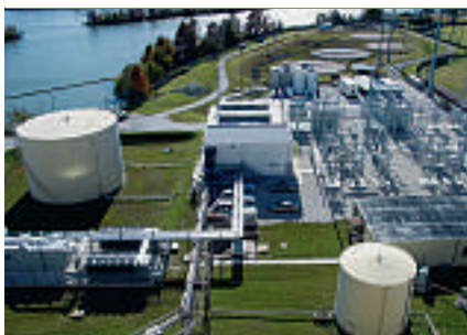
5 Austin Energy plant (Texas) with SVC Light® rated at ±95 MVar.
