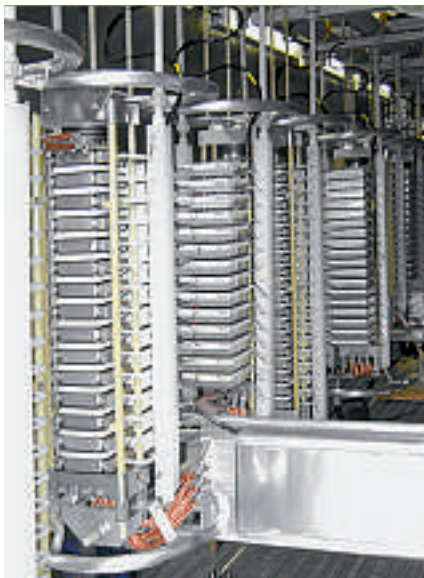
4 SVC Light valve assembly.
