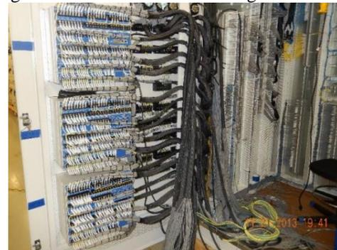
Figure 1 A data center low voltage compartment example showing conventional CT wiring for a bus differential
