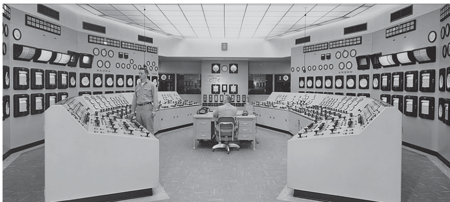
2 A control room from the 1950s
