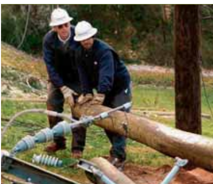
2 Hurricane Damage to electricity poles
