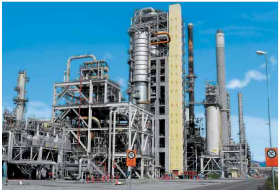
A modern and complex oil and gas process plant
