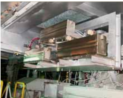
6 Hot Gauge platform with ABB EM Stabilizer magnets
