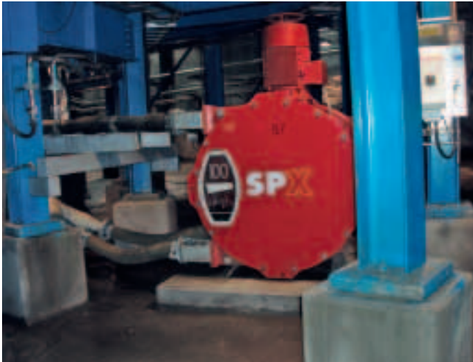
Bredel SPX100 high-pressure hose pump below one of the thickeners. Its inner hose diameter is 100 mm, minimum starting torque 4,650 Nm and capacity per revolution is 40 litres. It offers a maximum flow rate of 72,000 litres/h (continuous) and 108,000 litres/h (intermittent)
