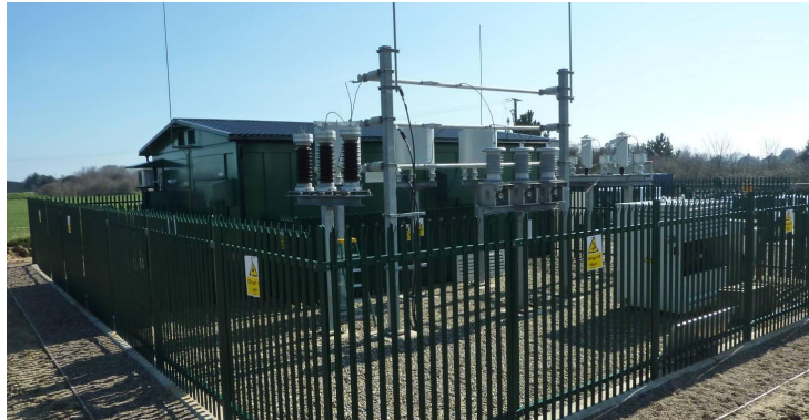
Fig. 9: DynaPeaQ installation, Norfolk, UK
