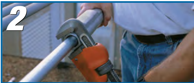
With a wrench, tighten the gland nut to compress the Teflon packing, creating a raintight seal around the conduit.
