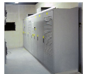
View of the cane mill (862 kW) and ACS1000 controlling the cane mill at Santa Matilde mill of Compañía Azucarera Hondureña S.A.
