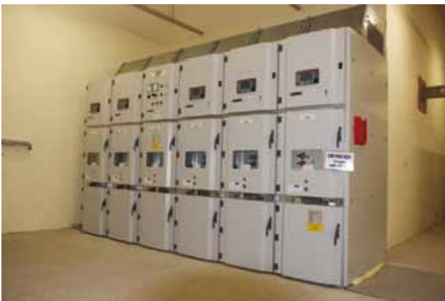
Medium voltage distribution system.
