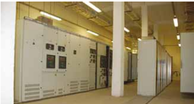
Low voltage distribution system and motor control centres.
