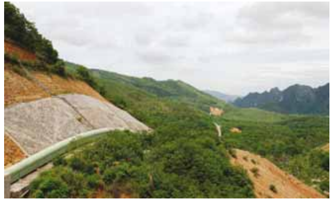
7.5 km long belt conveyor from the crusher to the storage area.
