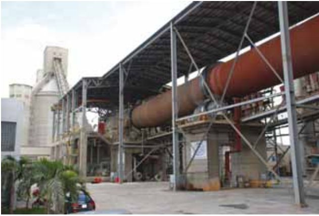
The kiln at the Cam Pha Cement plant.
