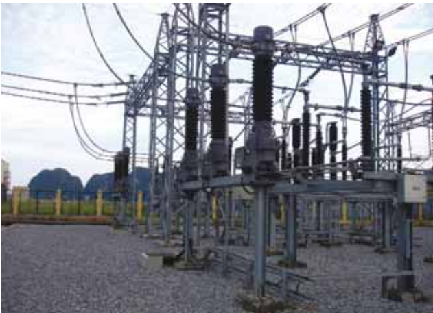
High voltage distribution system.
