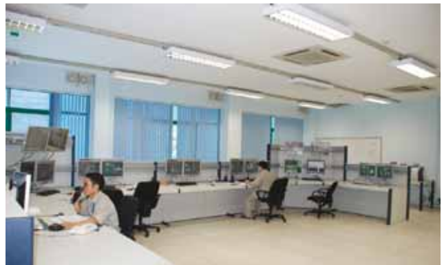
Central control room at Cam Pha.
