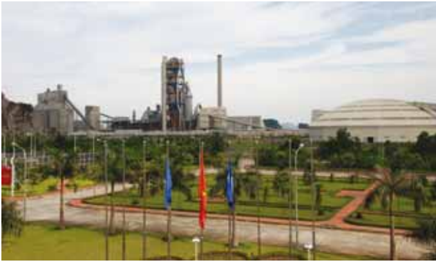
Cam Pha Cement plant.
