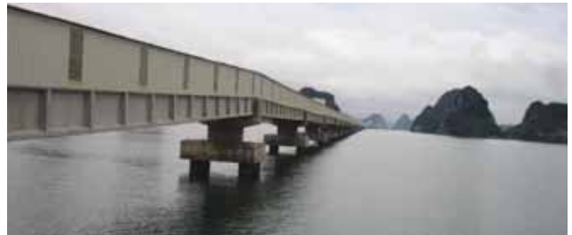
Long belt conveyor to ship loader and unloader.
