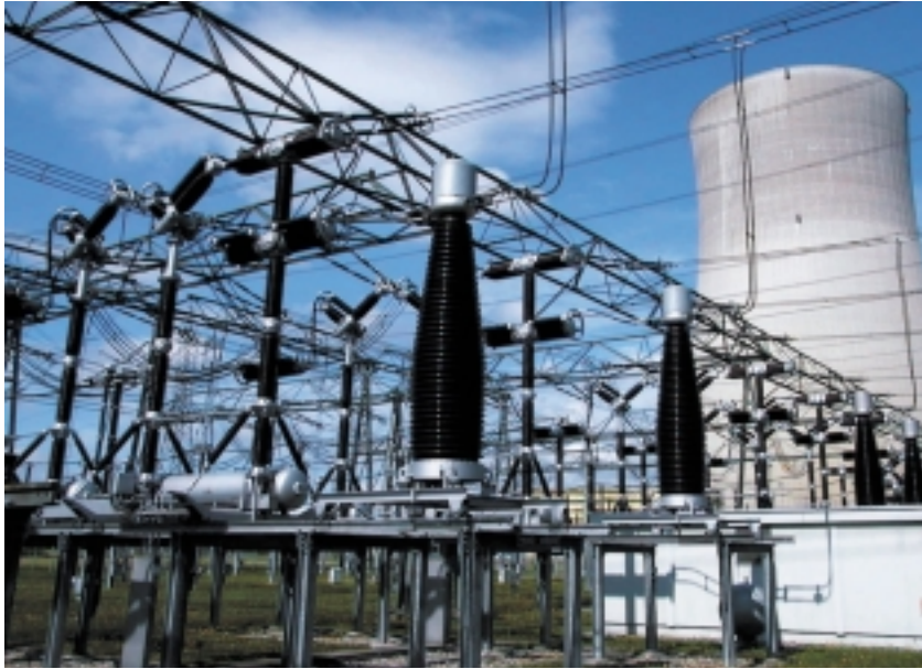
3 Power plant managers need to be able to compare assets within a plant and estimate their remaining life. Monitoring of the state of the process enables operators to schedule preventive maintenance and avoid costly downtime.
