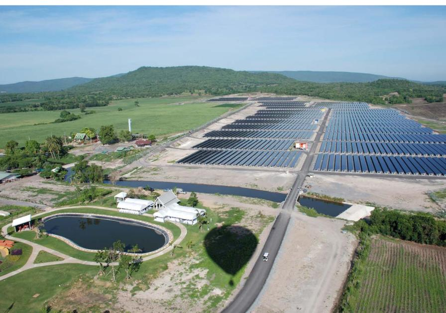
The Lopburi solar plant in Thailand is a 73 megawatt field of photovoltaic cells, covering an area around 250 football pitches. It delivers enough electricity to power 70,000 local households. The delivery of that power is managed with ABB's MicroSCADA Pro software, to ensure the greatest possible efficiency in generation and maintenance of the site.
