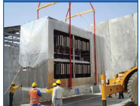
Placing the rectifier
