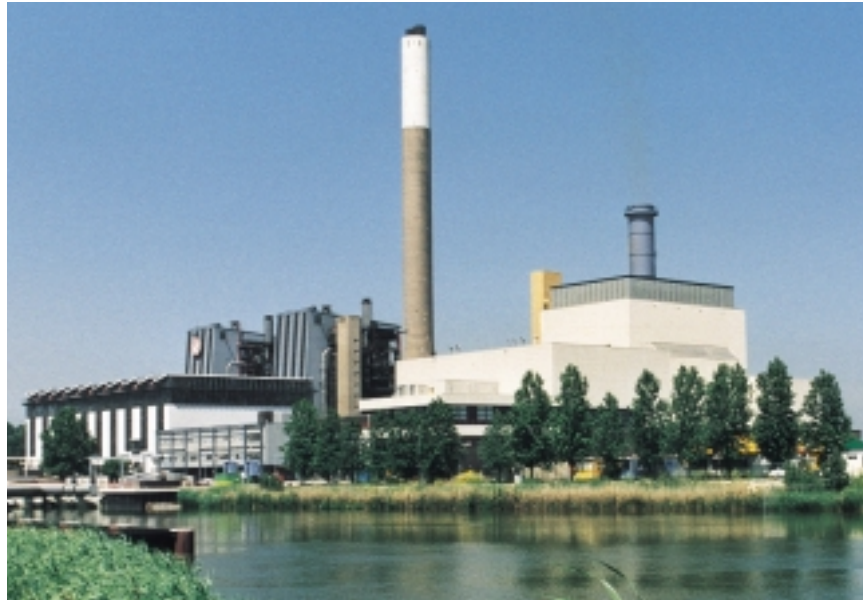
Diemen 33 combined cycle power plant in the Netherlands. This plant corresponds to a type E facility.
