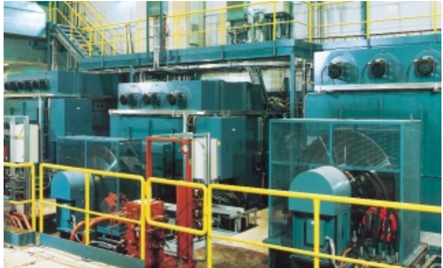
View of the three main drives delivered by ABB for the roll stand and coilers
