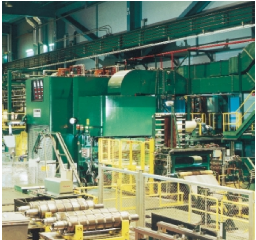
New cluster mill for cold-rolling stainless steel strip in the Tornio works of Outokumpu Polarit Oy, Finland. The mill is equipped with a global process control system that supervises production and controls the plant automation function.
