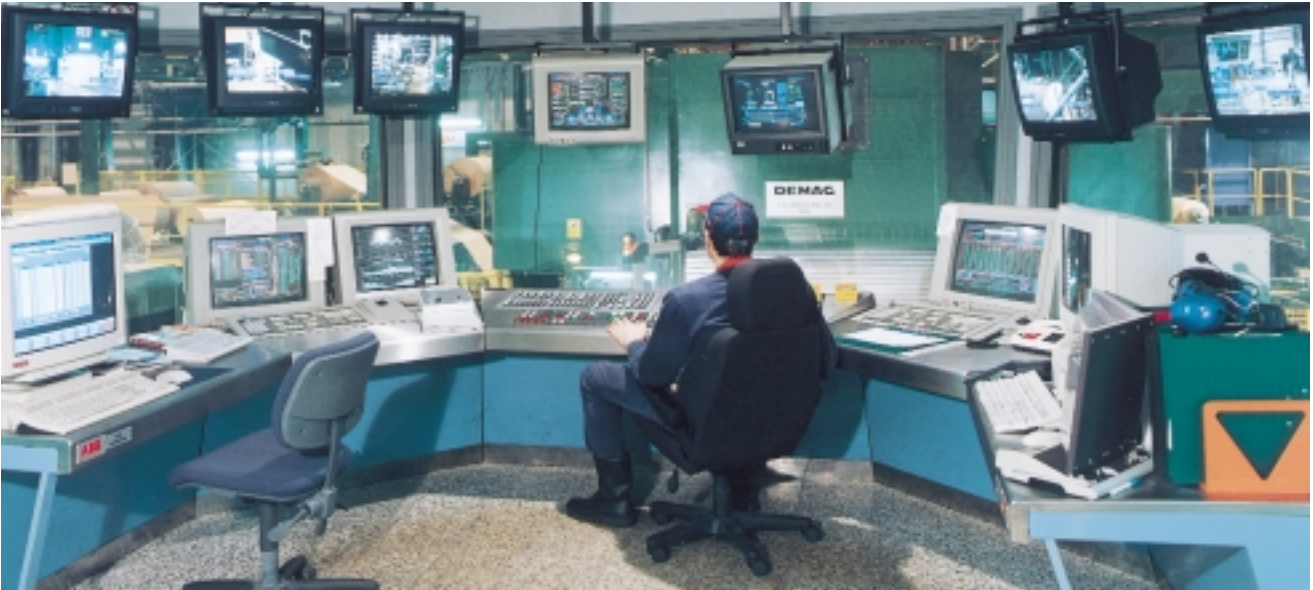
Main operator's desk
