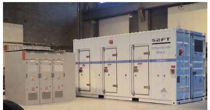
System at Letterly substation
