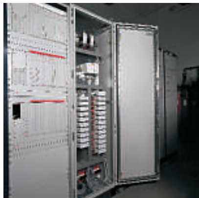
ControlIT AC 800M controller and S800 I/O units in the Kemira plant
