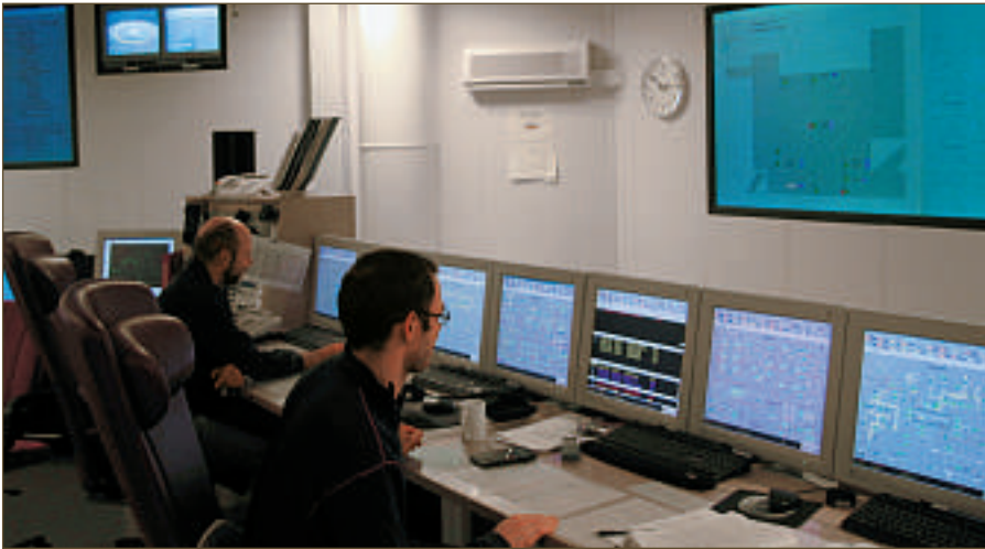
Operator stations and one of the large screens in the Grane control room
