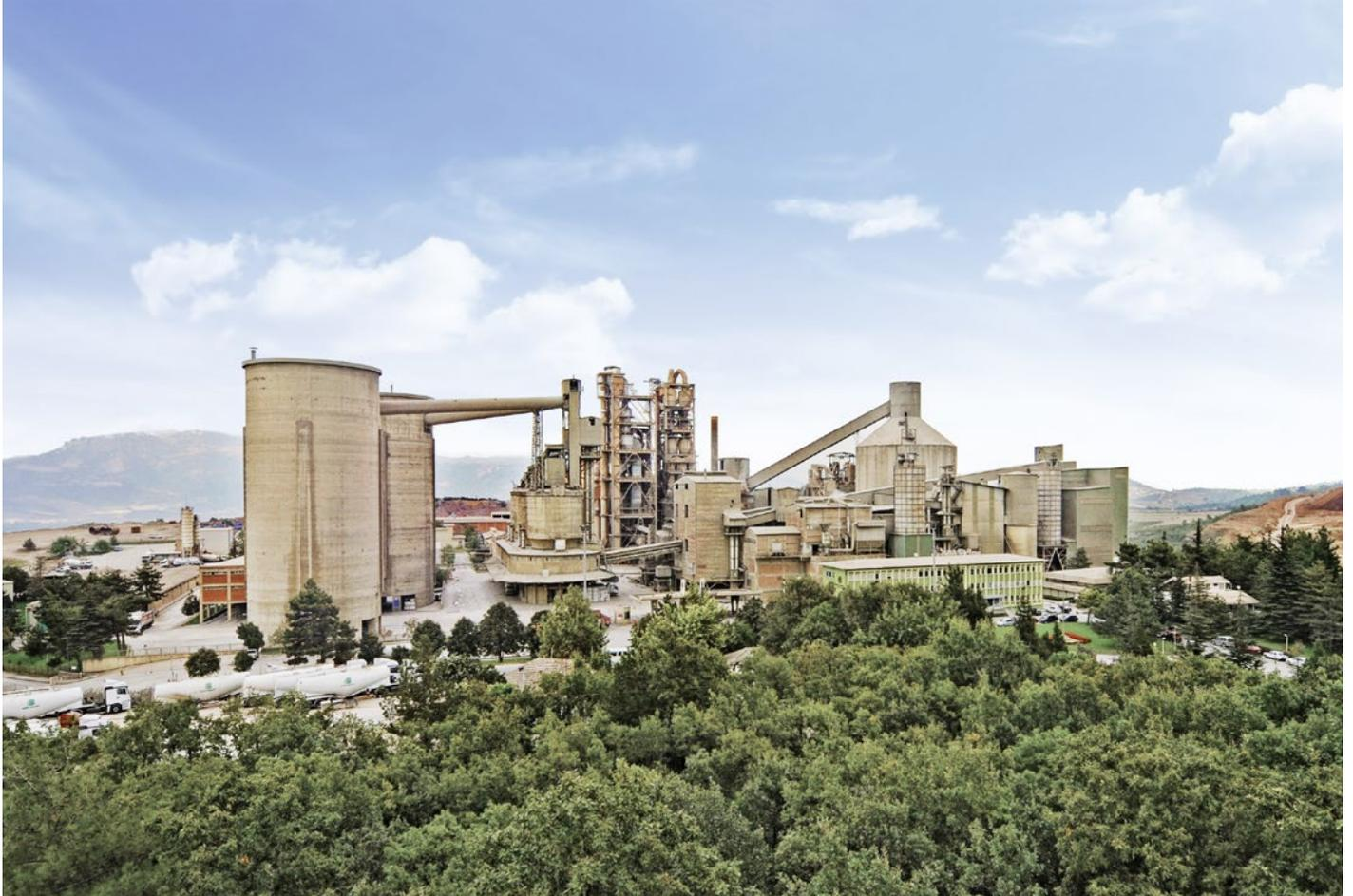
ABB's Expert Optimizer (EO) project, carried out on line 1 at the plant, provides advanced kiln control and stability. The line consists of a 50 meter rotary kiln with a 5-stage preheater and an in-line calciner. Plant operators welcomed the new system as it quickly showed benefits, including utilization factors higher than 90% at the beginning of the commission.
