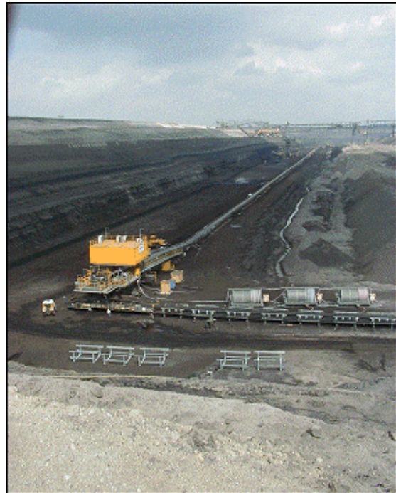
Fig. 1: View of a coal conveyor
