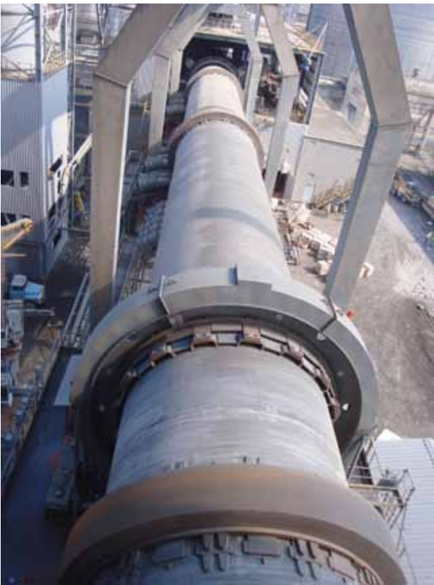
Kiln line no. 7 at Podilsky Cement.
