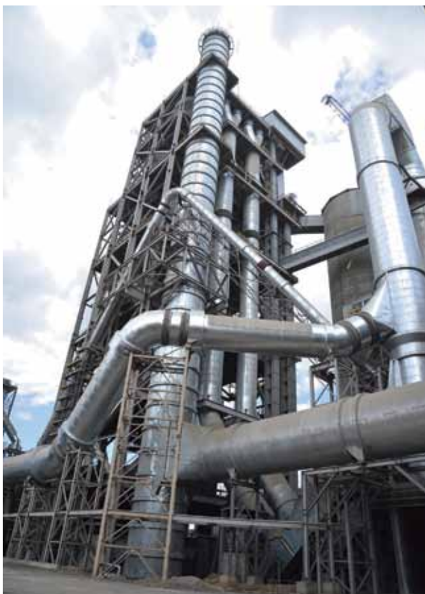
The preheater tower.
