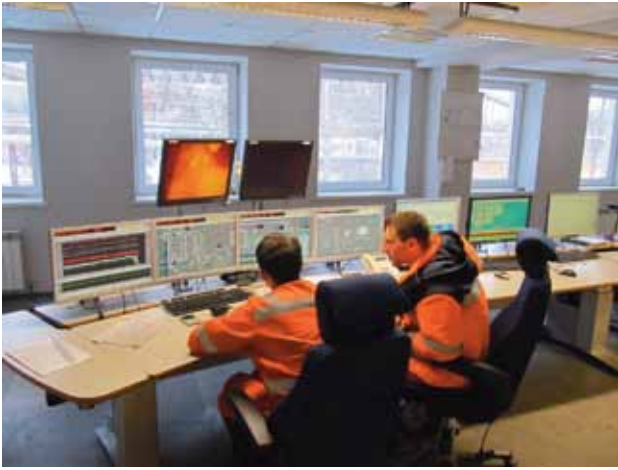
New central control room (CCR).
